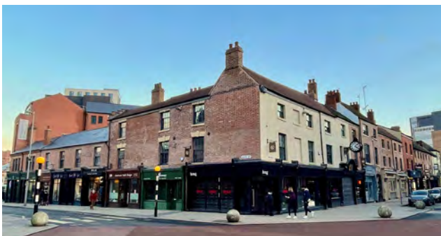
Coventry's The Burges before and after a £10m revitalisation scheme (Image: Google)
